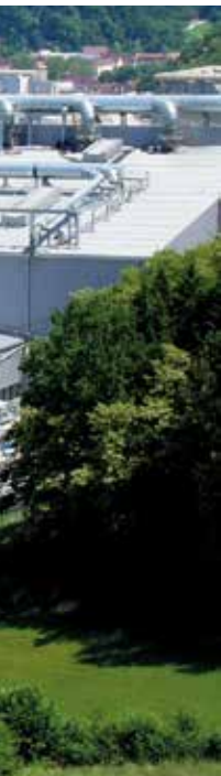
The new electric steel plant in Kapfenberg sets new standards in production quality, process reliability and environmental practice.
